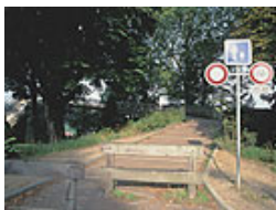
Entrance to the pedestrian bridge over the Seine.
