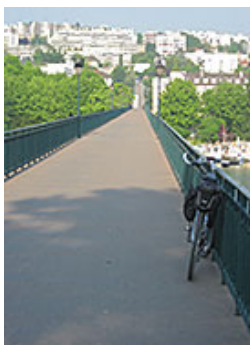
The pedestrian bridge.
